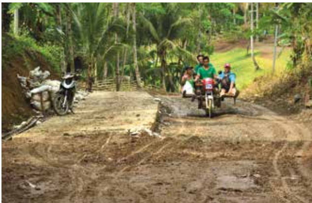
A farm-to-market road project in Santiago, Agusan Del Norte. Source: dar.gov.ph
