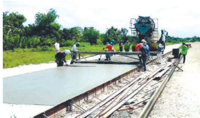
Construction of New Bacolod Economic Highway • Source: DPWH
