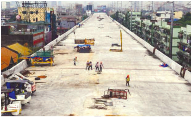
Skyway Stage 3 Ongoing Construction • Source: ABS-CBN News
