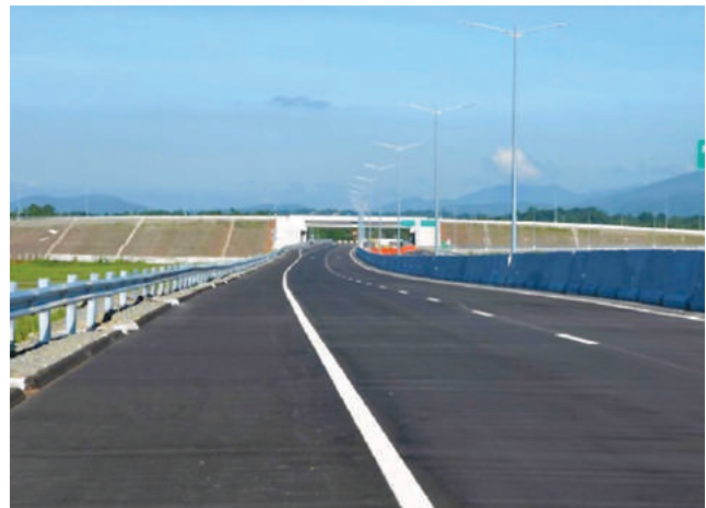
Tarlac-Pangasinan-La Union Expressway (TPLEX) • Source: Rappler
