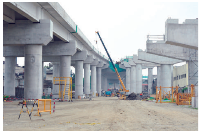
NLEX-Harbor Link Segment 10 Construction • Source: MNTC
